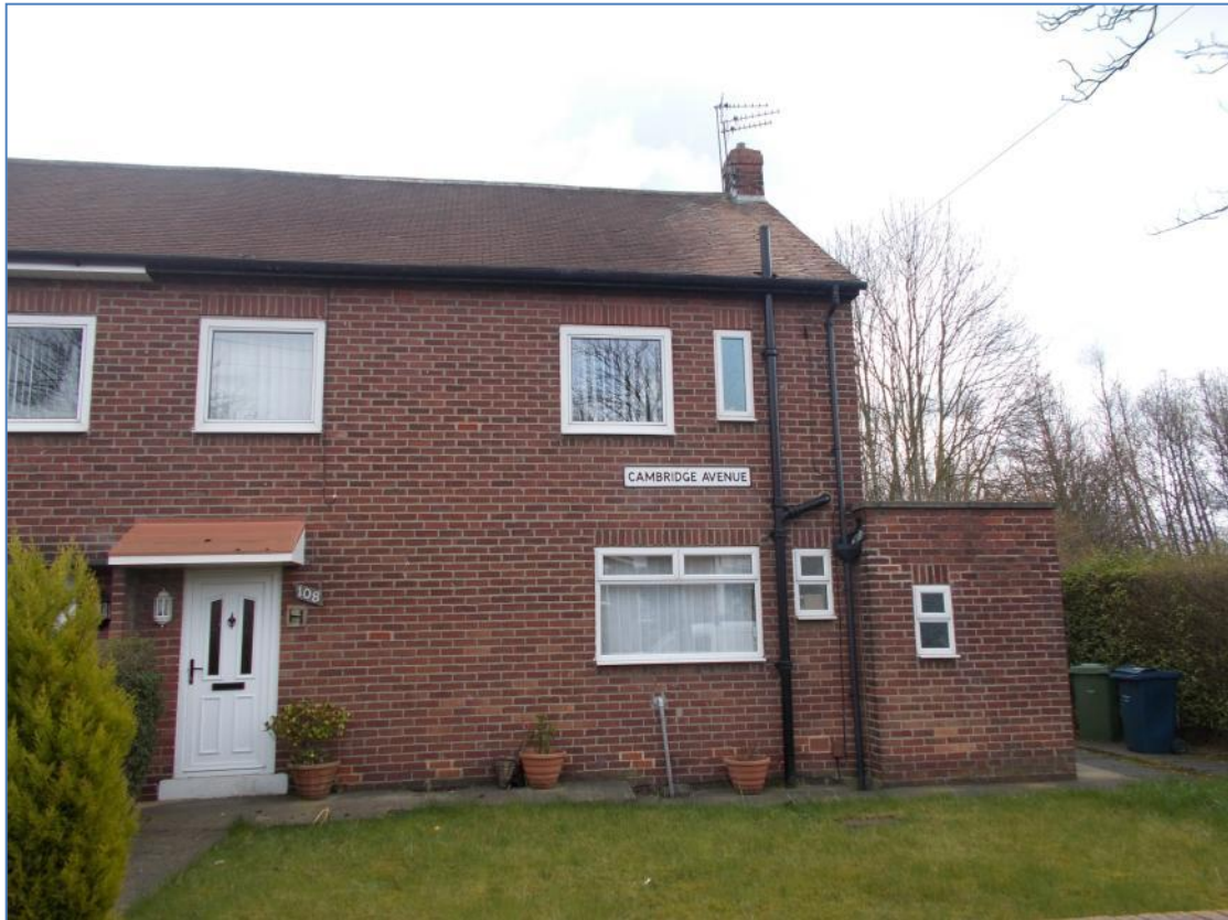
Photograph 1 – North-west elevation of 108 Cambridge Avenue.
